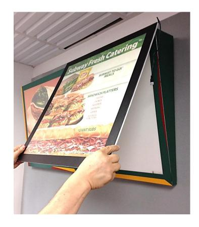
Carefully lift the unit – aligning it with your existing menu board. Place the top bracket on to the top of your existing hardware – making sure it's secure. Then slowly lower the entire unit over the face of your menu board. The high-powered magnets will "click" – holding it tightly.
